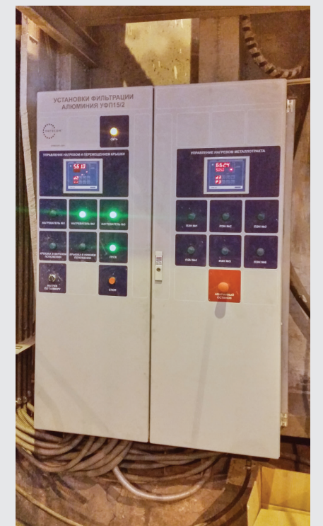
Ontecom's filter box electric cabinet
