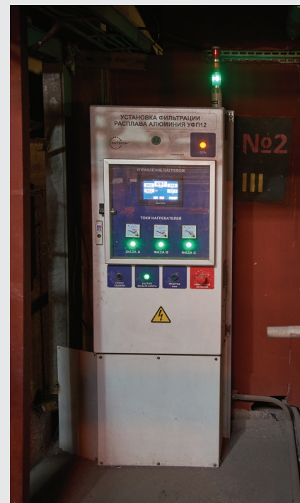
Ontecom's filter box control cabinet, PLC and HMI based
